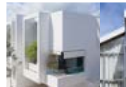
THE RESIDENCE BY ANDAMAN ASSET SOLUTION
